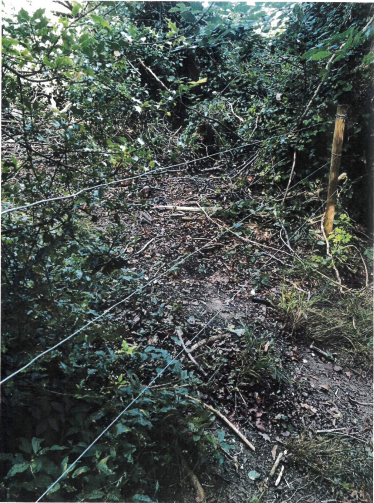
Fence repair Magpie Wood 17 August 2023
