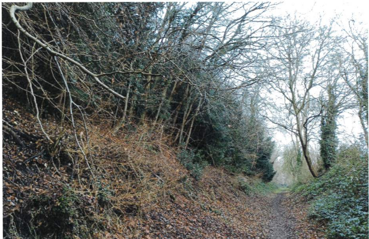
Photo 1 looking north-west from base of cutting with 15-20m high cutting face on left and circa 3m high face on right
