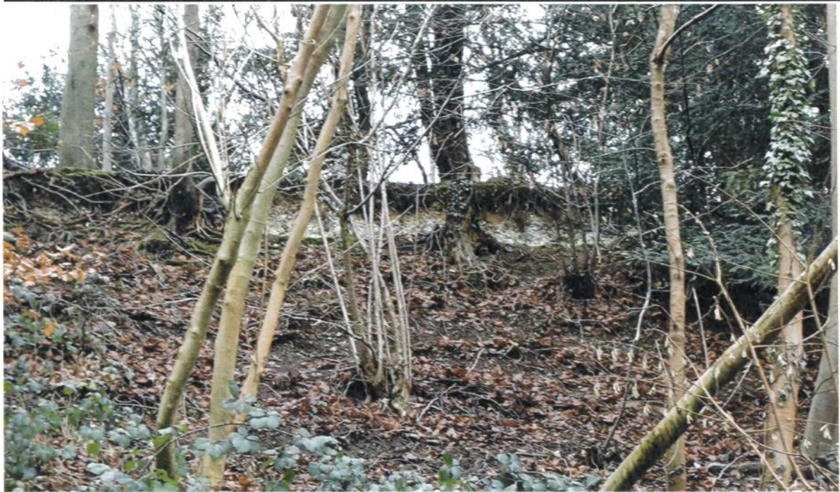
Photo 5 Near vertical backscarp at crest of cutting
