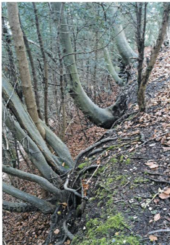
Photo 6 showing tree root systems partially stabilising backscarp at crest of cutting
