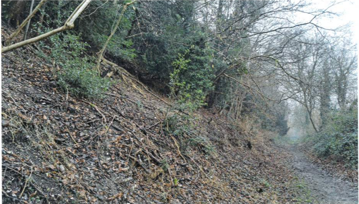
Photo 3 showing local accumulations of topsoil/subsoil on lower section of cutting face
