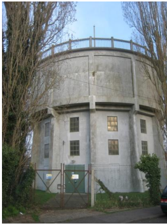
Current water tower in Georges Drive
